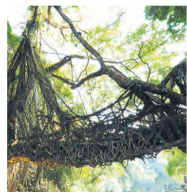
Roots Bridge in Mawlynnong, Meghalaya are devoid of any brick, steel or mortar
