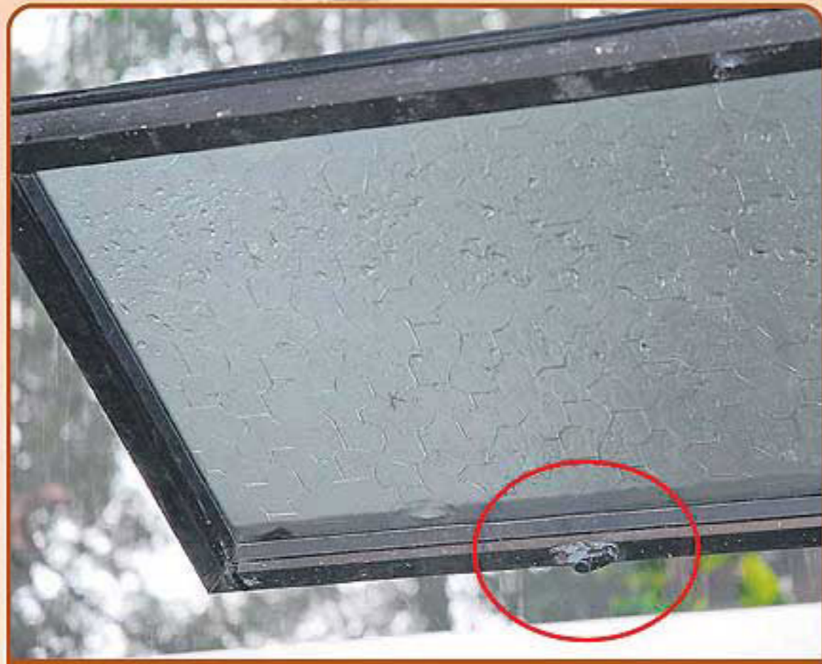
The window has two panels. Grilles were to have been installed but weren't because of a misunderstanding between the ISD and the vendor. When this was discovered, the centre's superintendent asked that the handle of the window be sawn off.
